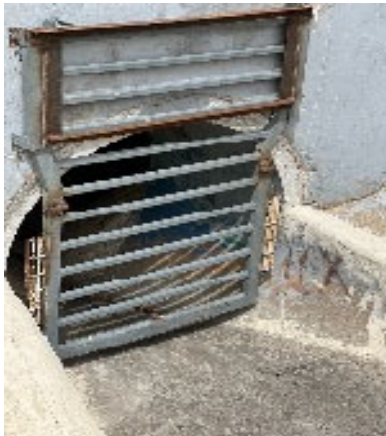
13 th Ditch Gate
